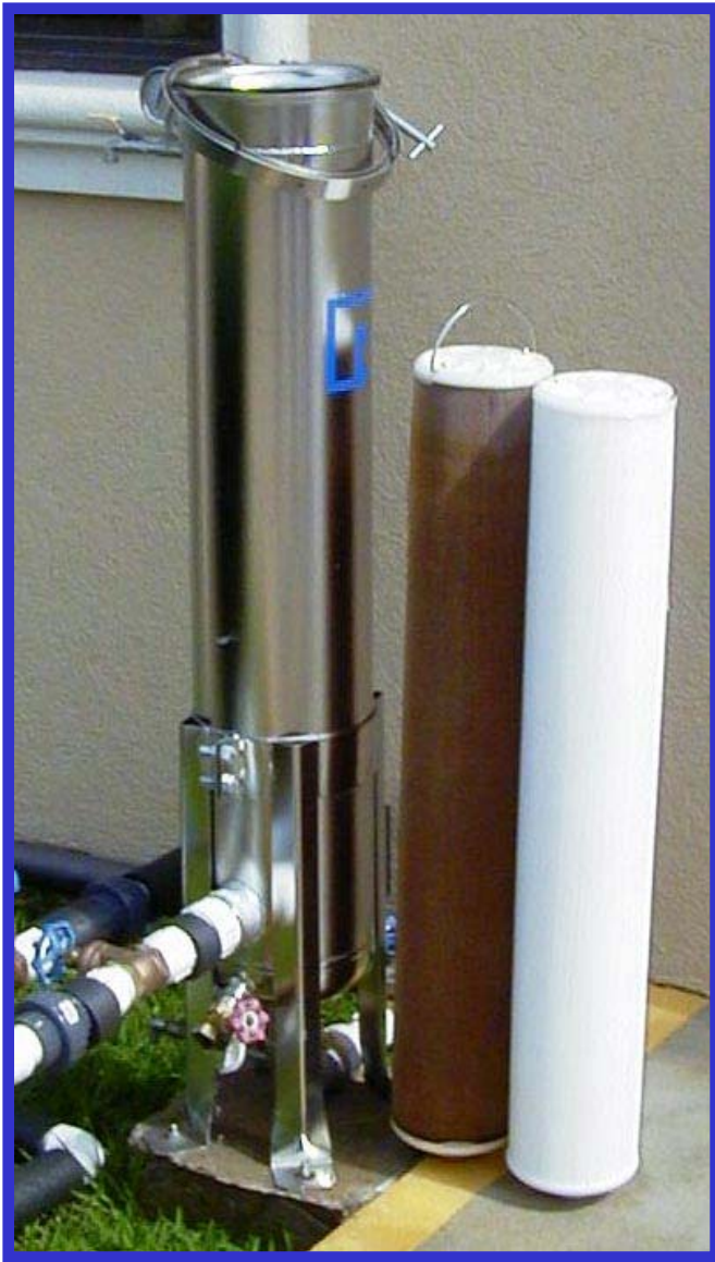
Used Filter on Left, New on Right.
